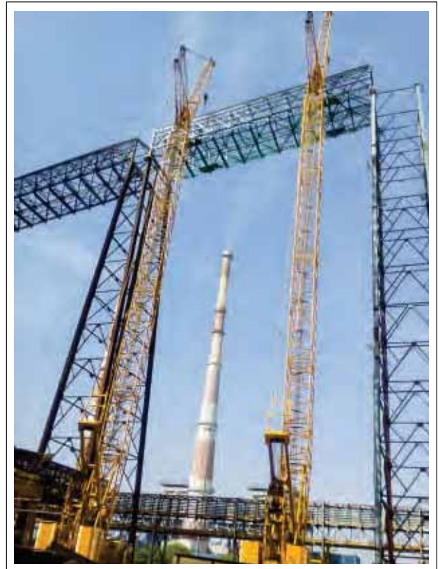
SANY SCC 2500C Crawler Cranes (Capacity 250MT) two nos. erecting 52MT in tandem with luffing configuration for Lanco Infratech Ltd, Korba, Chhattisgarh
