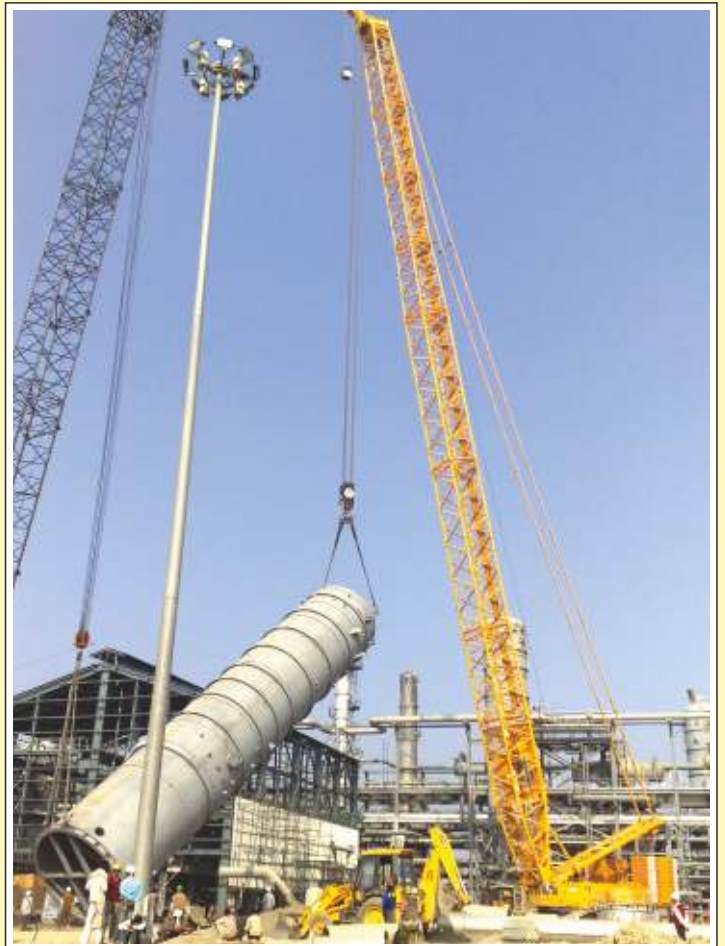
LIEBHERR LR 1400 - 2 Crawler Crane (Capacity 400 Ton) working at petrochemical plant in northern part of India
