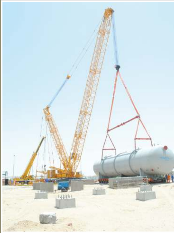
LIEBHERR LR 1400 - 2 Crawler Crane (Capacity 400 Ton) and LIEBHERR LTM 1100 - 1 Tyre Mounted Telescopic Crane (Capacity 100 Ton) working at refinery in western part of India
