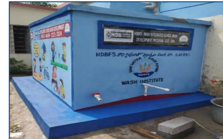
Safe Sanitation Complex, WASH
