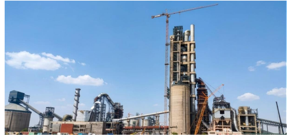
Nagaur IU – Pyro-processing and Clinker Storage
