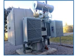
Shunt Reactors
