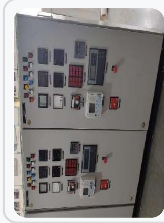
Control & Relay Panels (CRP) up to 33kV
