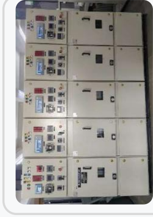
11kV Vacuum Contactor Panel
