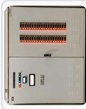
Power Distribution Unit (PDU)
